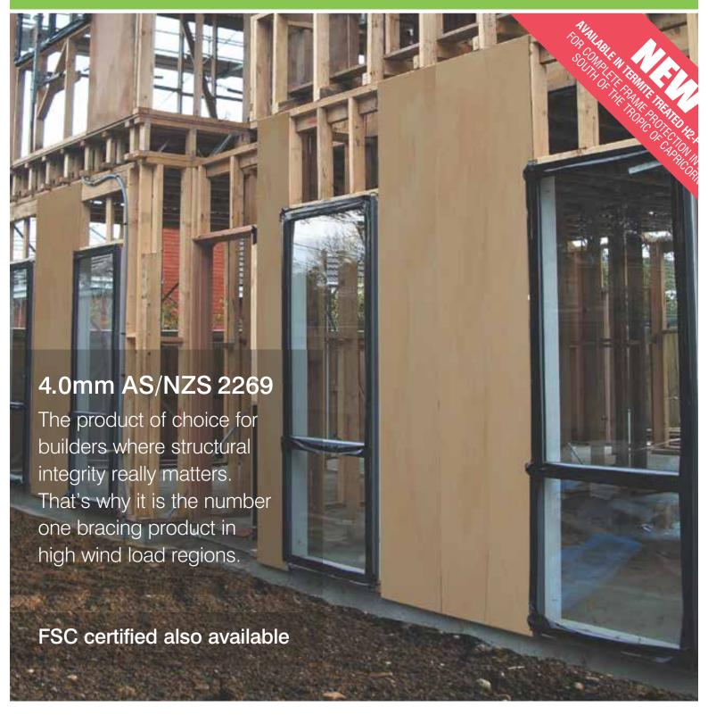
The Gunnersen bracing range now includes 4.0mm thick hardwood plybrace panels that can achieve up to 7.5Kn per metre racking resistance when installed in accordance with the AS1684.2-2006 framing code.
