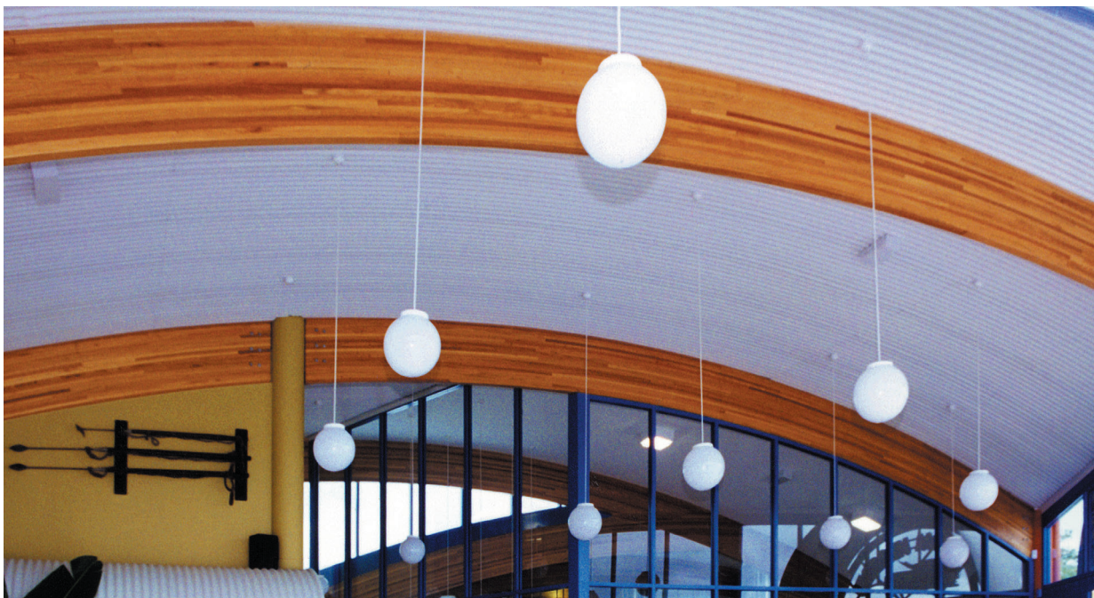
Figure 6: Glue laminated engineered timber products
