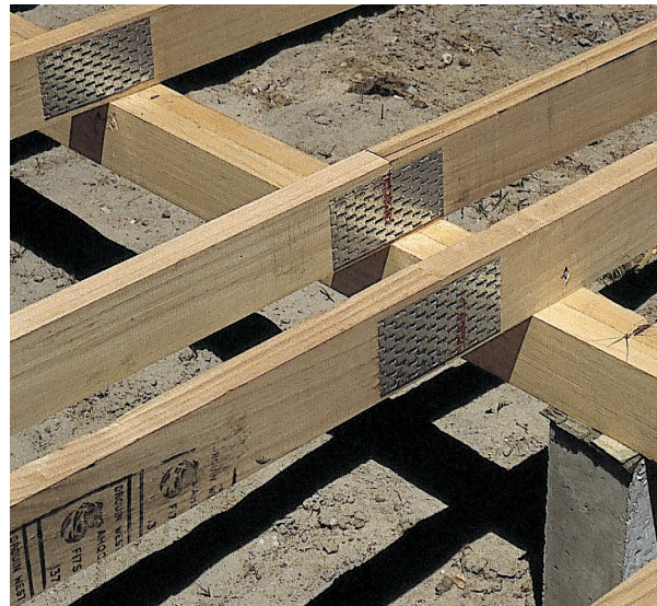
Figure 5: Nail plated kiln dried, dressed products
